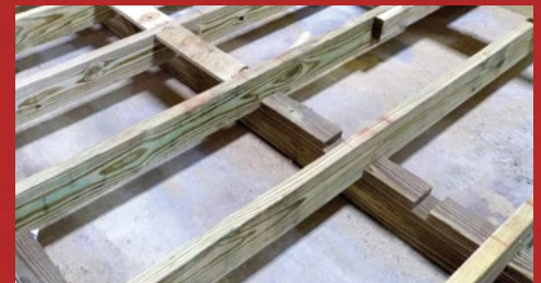
12" On-Center Floor Joists 16" OC is Standard
