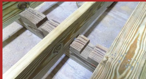
2x6 Pressure Treated Joists 2x4 are Standard
